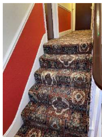
Half Landing Stairs to Rooms 10 & 11.
